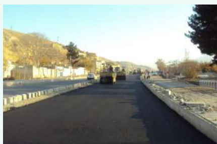
51 km Doshi-Pol-E-Khomri Existing Road Rehabilitation, Afghanistan
