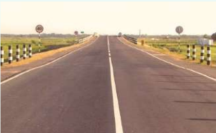
61 km Sylhet-Tamabil-Jaflong Road Rehabilitation, Bangladesh
