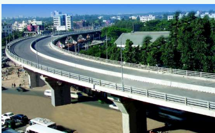
Mohakhali Flyover at Dhaka (Dhaka Urban Transport Project), Bangladesh
