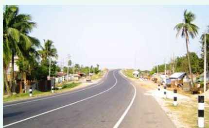
223 km long Dhaka-Sylhet Road Rehabilitation, Bangladesh
