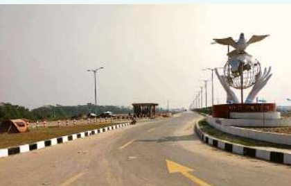
4-Lane Rajapara-Payra Port Connecting Road, Bangladesh
