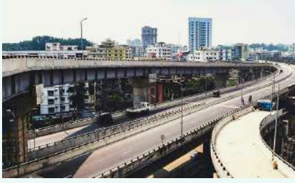
Muradpur Flyover at GEC Junction Chittagong, Bangladesh
