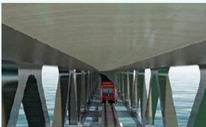
Padma Multi Purpose Bridge (PMPB) Railway Link, Bangladesh
