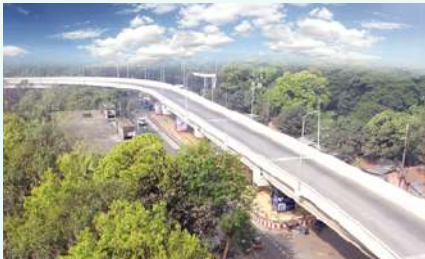
Kadamtali Junction Flyover at Chittagong, Bangladesh
