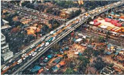
Railway Overpass & Connecting Road at Bijoy Sharani Dhaka, Bangladesh
